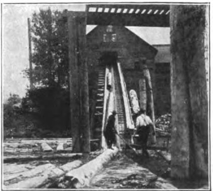
HOISTING LOGS TO MILL
